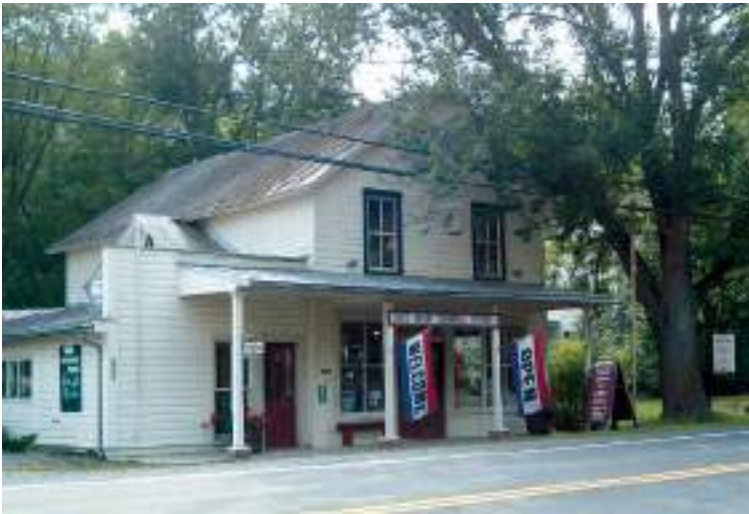
The Lost River General Store, still standing as it did when James Ward Wood spent time there while recovering from his wounded leg in the summer of 1865. The store is located at 6993 State Road 259, Lost River, West Virginia.
