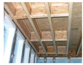
Install blocking and bracing between joists according to the instructions of the Builder Guideline Booklet.
