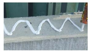
Construction adhesive is recommended between the Bond Beam and the Sill Plate (a 2x10 Sill Plate is recommended).
