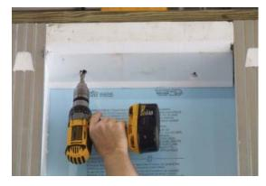
When holes are provided in the concrete Bond Beam, drill through the sill plate from below (Xi Wall System).
