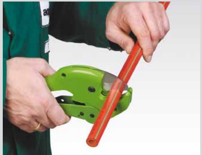
Cutting of the pipe
