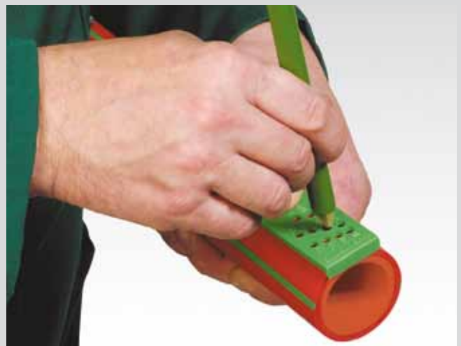
Marking of the welding depth
