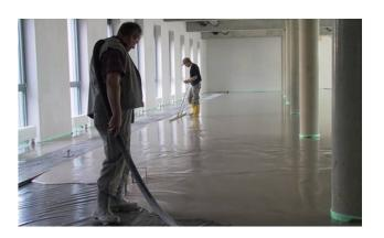
**Shrinkage** – Ultraflo has virtually no drying shrinkage. Movement joints need only be considered where the floor exceeds 1000m<sup>2</sup>, or where the floor becomes elongated and an aspect ration of 1:6 is exceeded. Movement joints should also be considered across doorways and when used with under-floor heating systems, movement joints should be considered between different heating zones.
