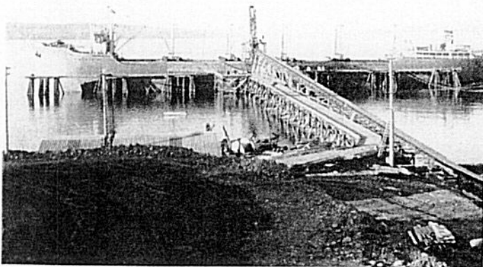
Ship loading facility, Port McNeill
