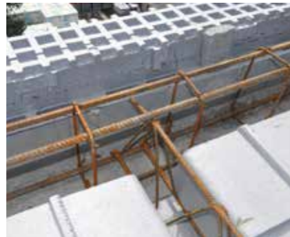
The MP element makes it possible to place reinforcement of the ring beam within the wall axis and floor support.
