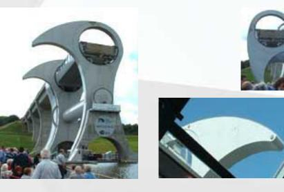
Wheel is powered by 10 hydraulic motors that turn the two caissons, each of which may accommodate up to four 20m long boats at any one time. Despite the scale of this power, each turn of The Wheel uses virtually no water and the same energy as just two boiling kettles.
