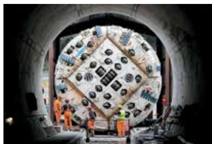
Boring the world’s longest rail tunnel.
