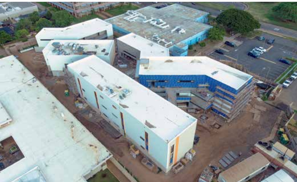
Swinerton is adding five new classrooms at Campbell High School.
