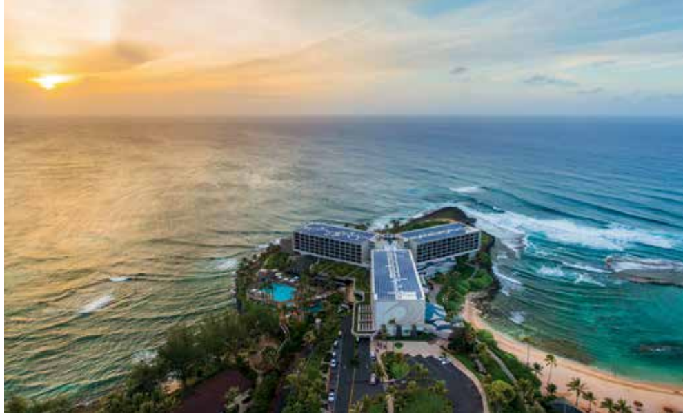
Swinerton is beginning a two-year renovation at Turtle Bay Resort.
