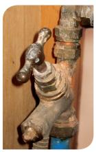
Your stop tap is usually located under the kitchen sink or in a connecting garage. It is important to know where it is and to check that it is working properly, in case you ever have to shut off your water in an emergency. If it is not working, we recommend that you call a plumber.
