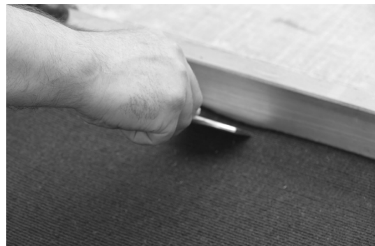
Knock down protruding ends with the stair iron
