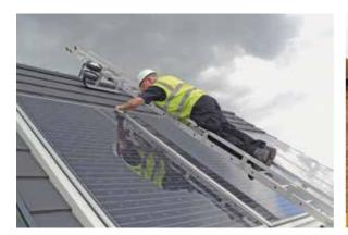
The Solar Ladder offers a safe, practical way of working when installing or maintaining solar panels. The bridging ladder provides 23cm clearance from the roof to the underside of the stile and up to 4.6m free span over the roof. The ladder is simply rolled up the roof on its soft rubber wheels and then flipped 90° into position on the roof. The ladder can also be easily traversed along the ridge with the use of special wheels fitted to the roof hooks.
