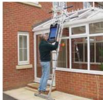
The Easi-Dec Conservatory Roof Access System is a specifically designed two piece system for accessing conservatory roofs, or any glazed roof, for cleaning and maintenance purposes.
