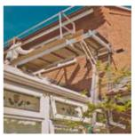
**End Support Frame:** This single leg support is ideal for where restricted access precludes use of the standard 2m Dec, such as over boundaries or projecting structures.
