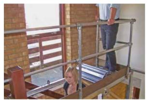
Walk Thru Stairwell Access has been designed as a safe solution to stairwell maintenance which is traditionally undertaken using boards and step ladders. The system provides users with a stable working platform above a staircase, whilst still allowing access up the stairs to the first floor. This is achieved by simply rolling back the aluminium slatted decking as required.
