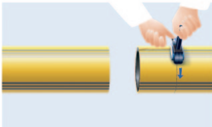
Fig. 2.21 Removal of the protective coating with the egeplast M10 peeling tool
