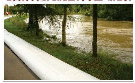
The system consists of two sleeves. Up to 10 m of on a possibility needs 2-3 people hydrant hose, floating pumps e.g. Niagara Falls, and water. filled time of one section is about 4-5 min, depending on the pump capacity. Working dimensions one section after filling with water:
