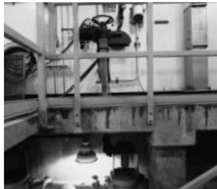
16" Cam-Centric® plug valve with extension stem and motor actuator.
