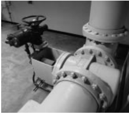
18" Cam-Centric® plug valve with motor actuator.
