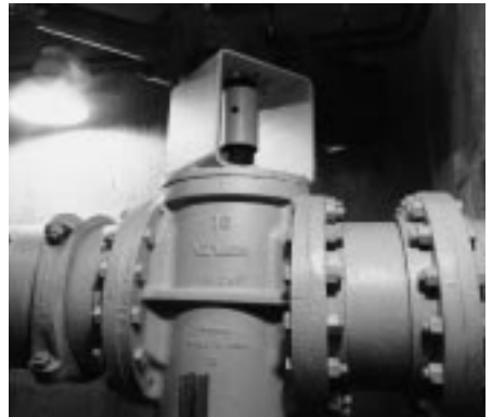
16" Cam-Centric® plug valve. Cylinder actuated with hydraulic, manual override.
