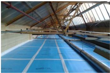
When removing a fragile roof or glazing it is critical that the Scaffolding Boarded platform is fully sealed and protected. This prevents any dust entering into the working environment below and also allows for an effective cleaning operation to be carried out before the Crash Deck structure is dismantled.
