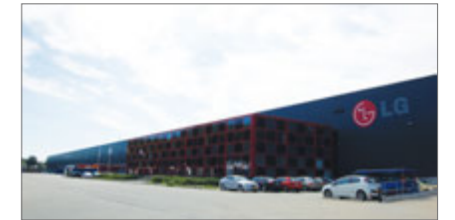
European Air Conditioning Distribution Center
